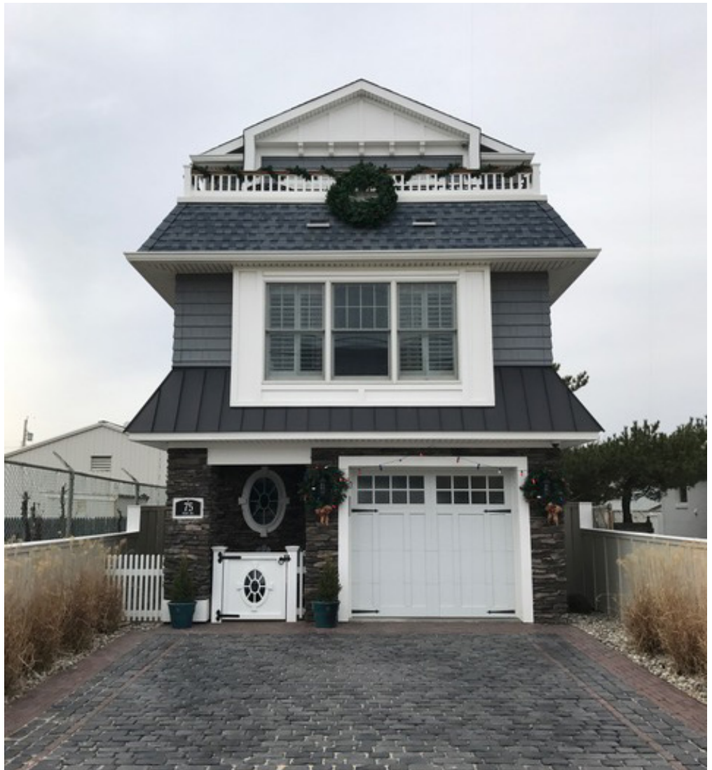
At left: The original beach bungalow in Manasquan before it was torn down by Atlantic Modular Builders to make way for a three-level beach house. Just above is the house after its big make-over.
