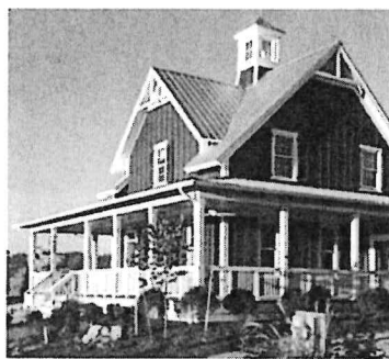
Country Living magazine's House of the Year in 2010 was this 1,607-square-foot modular cottage designed by New World Home. It was first shown in New York City and then moved to Crystal Springs Resort Hardystown.
