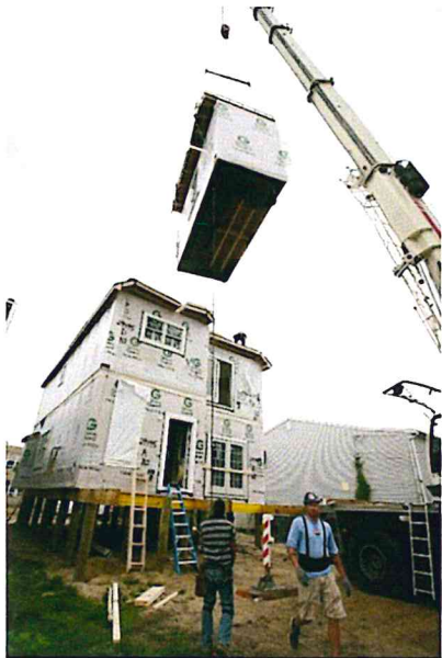
A crane places a section of a modular home being built to replace one destroyed by Hurricane Sandy in Manasquan.
